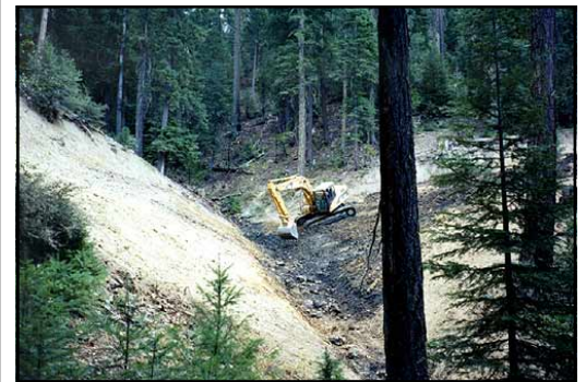
Excavated Stream Crossing
