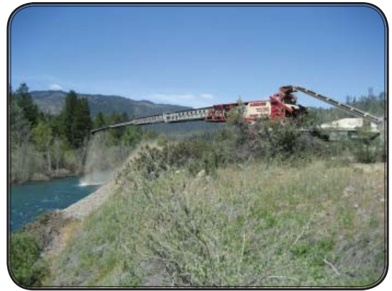
Conveyor system adding gravel at the Sawmill site, upper Trinity River.
