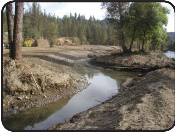
Newly constructed side channel at Indian Creek restoration site.
