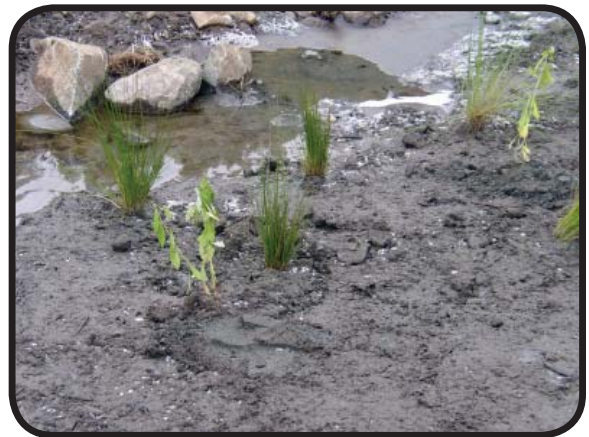
Deeply planted live stake cuttings of Cottonwood and Willow along bank at Sven site.
