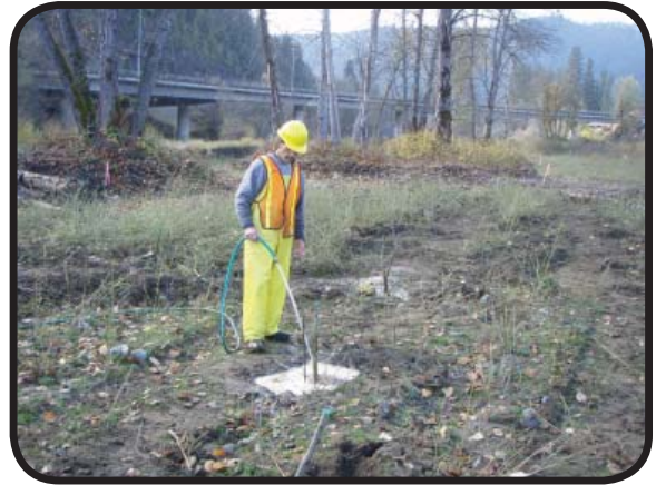
Watering fresh "pole" plantings to increase root to soil contact.
