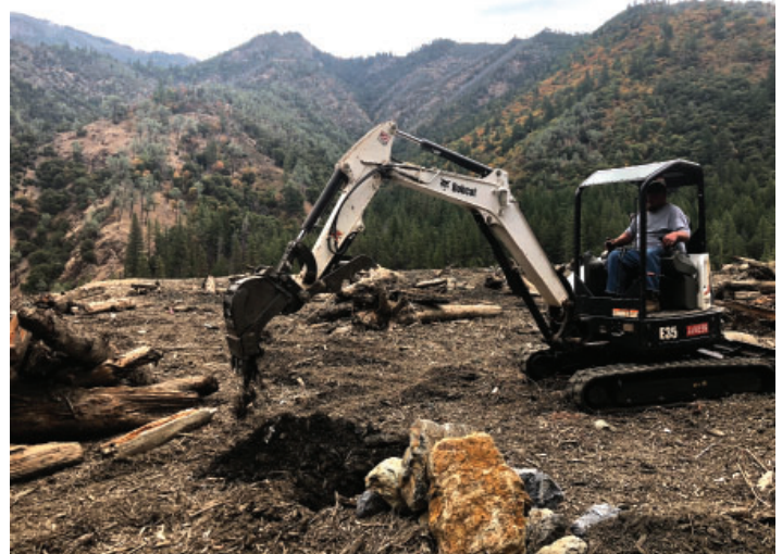
Digging holes for planting native trees and shrubs
