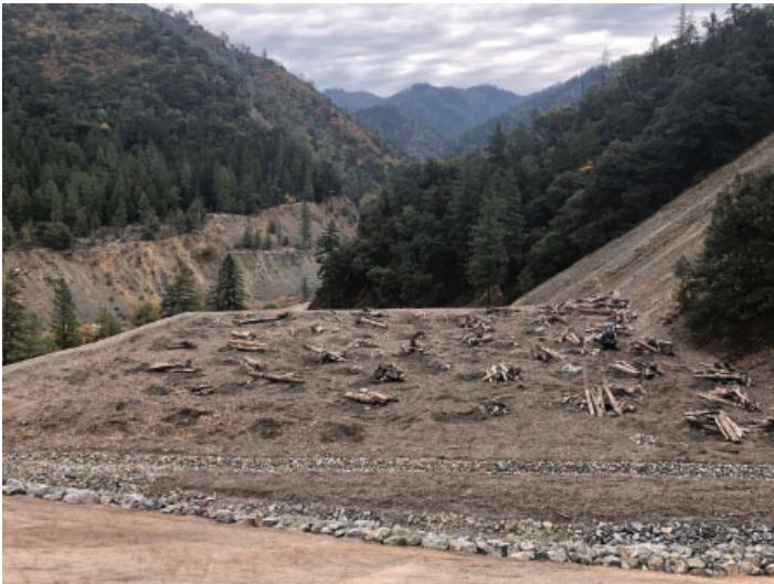
Revegetation at Big French Creek disposal site
