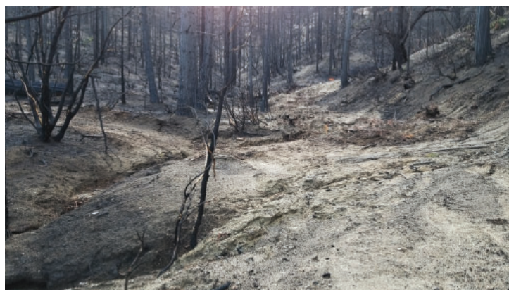
Stream crossing erosion on Mainline Spur A Road
