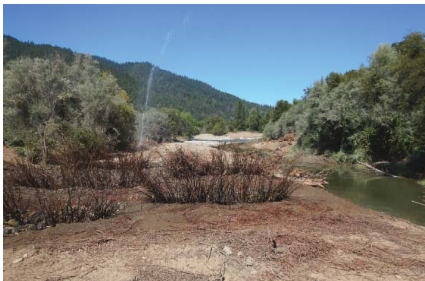
Newly placed willow trenches at the 2019 Chapman Ranch channel rehabilitation project near Junction City.
